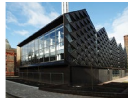
Figure 11.6 University of Liverpool Heating Infrastructure, Levitt Bernstein
